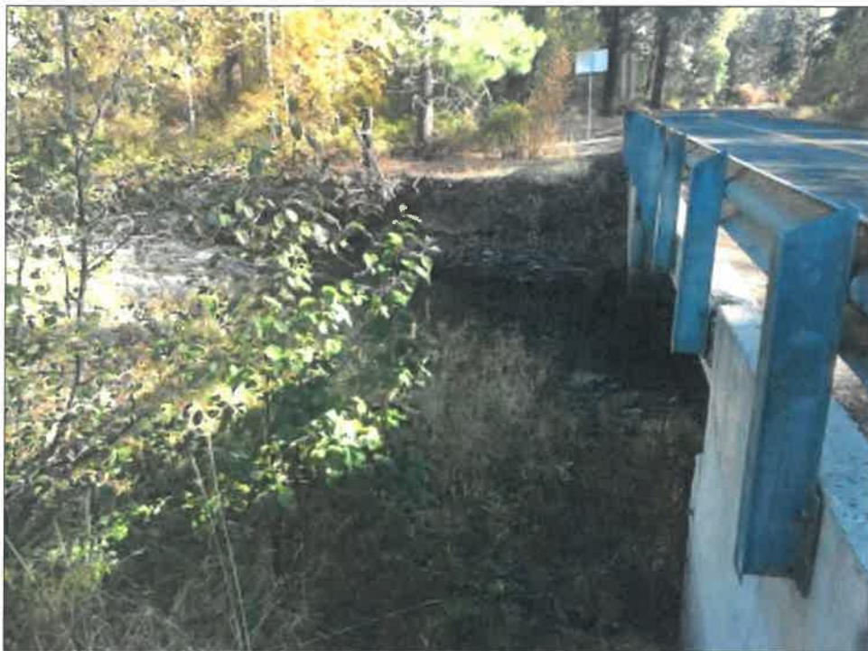
Photo 7. Vegetation on north side of bridge.
