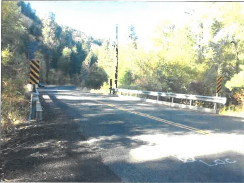
Photo 1. Manastash Road Bridge.
